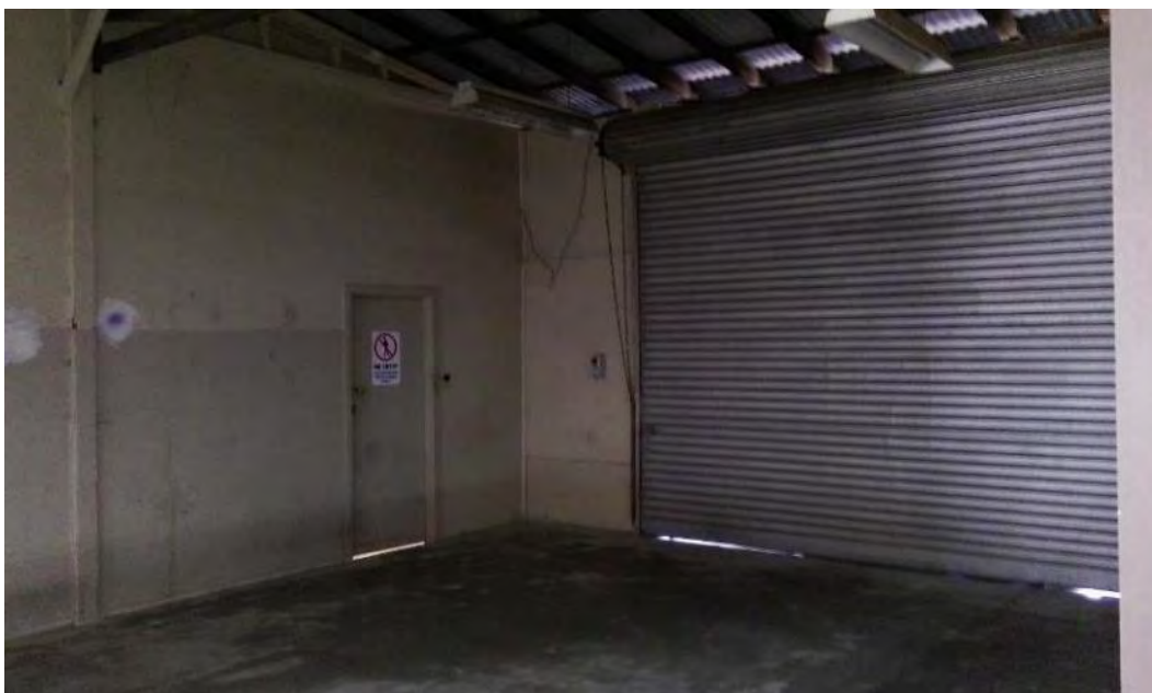
JobQuest storage space before converted to training room
